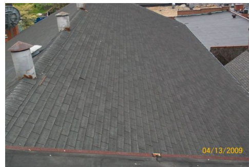
Roof Area 2 Facing South
