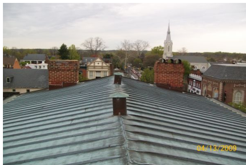
Roof Area 1 facing West
