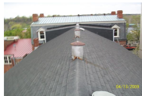
Roof Area 2 Facing North
