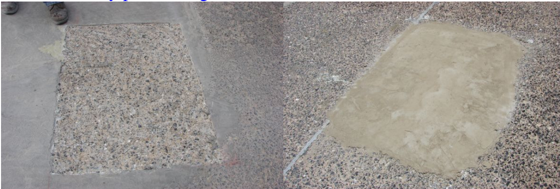
The area is cut & removed
